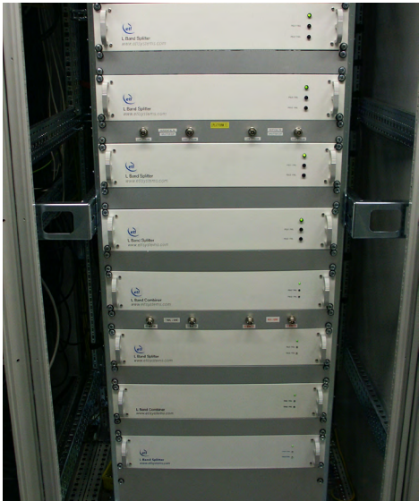
ETL's RF Splitters at a ground station
